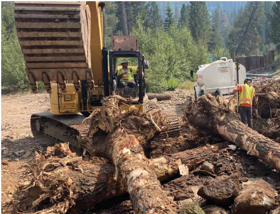
Above: Logs and boulders embedded in the streambank will protect against erosion and provide aquatic habitat. Michele Prestowitz Right: Bear Creek location: 10 miles South of Truckee or 3.5 miles north of Tahoe City on the north side of Alpine Meadows Road.
